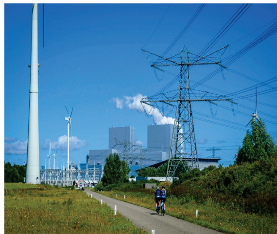
Windpark RWE, Eemshaven
