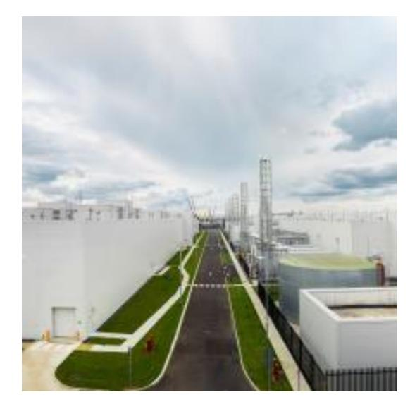
Microsoft uses air cooling in our Datacenters in the Netherlands. This method uses **outside air instead of water** for cooling at temperatures below 25 degrees Celsius, reducing water use to less than five percent of the year.
